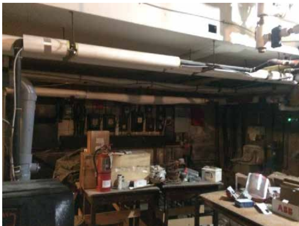
Photograph 11. View of the mechanical room, located in the basement of the church
