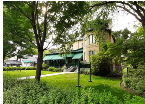
Figure 20, 21, & 22: View of Laurier House National Historic Site with rendered views illustrating the views from the front veranda suggest a minimum impact. Source Linebox 2023.
