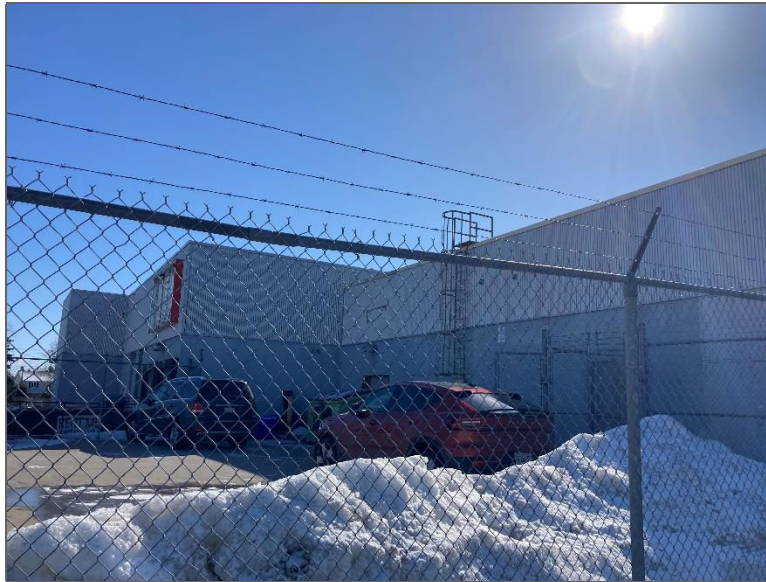
Photo 1 – Site Building (north elevation).
