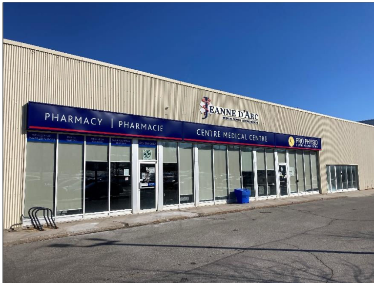
Photo 2 – Site Building (south elevation).
