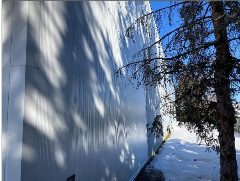
Photo 3 – Site Building (east elevation).
