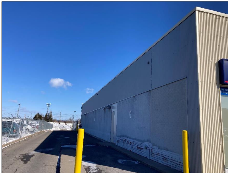
Photo 4 – Site Building (west elevation).
