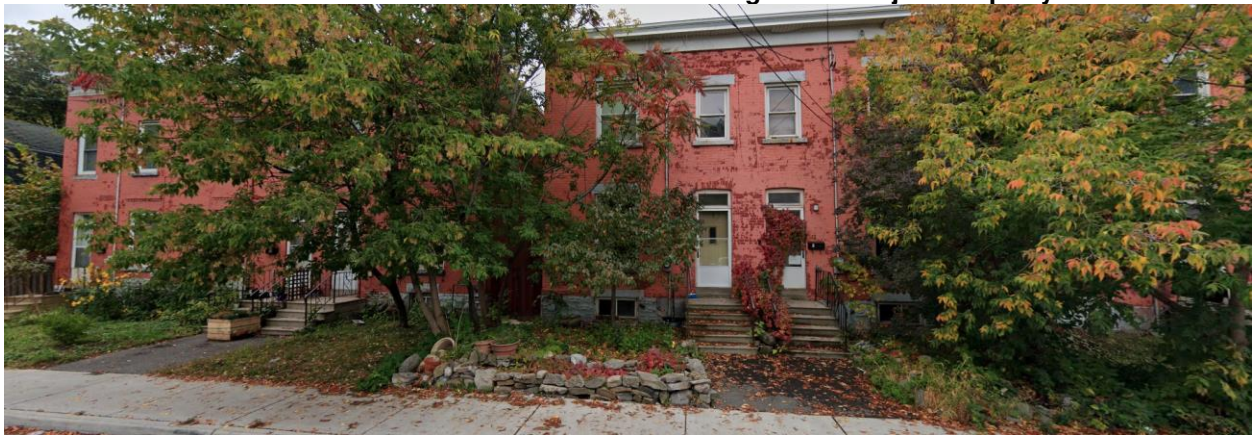
Figure 2: Subject Property from the Street
