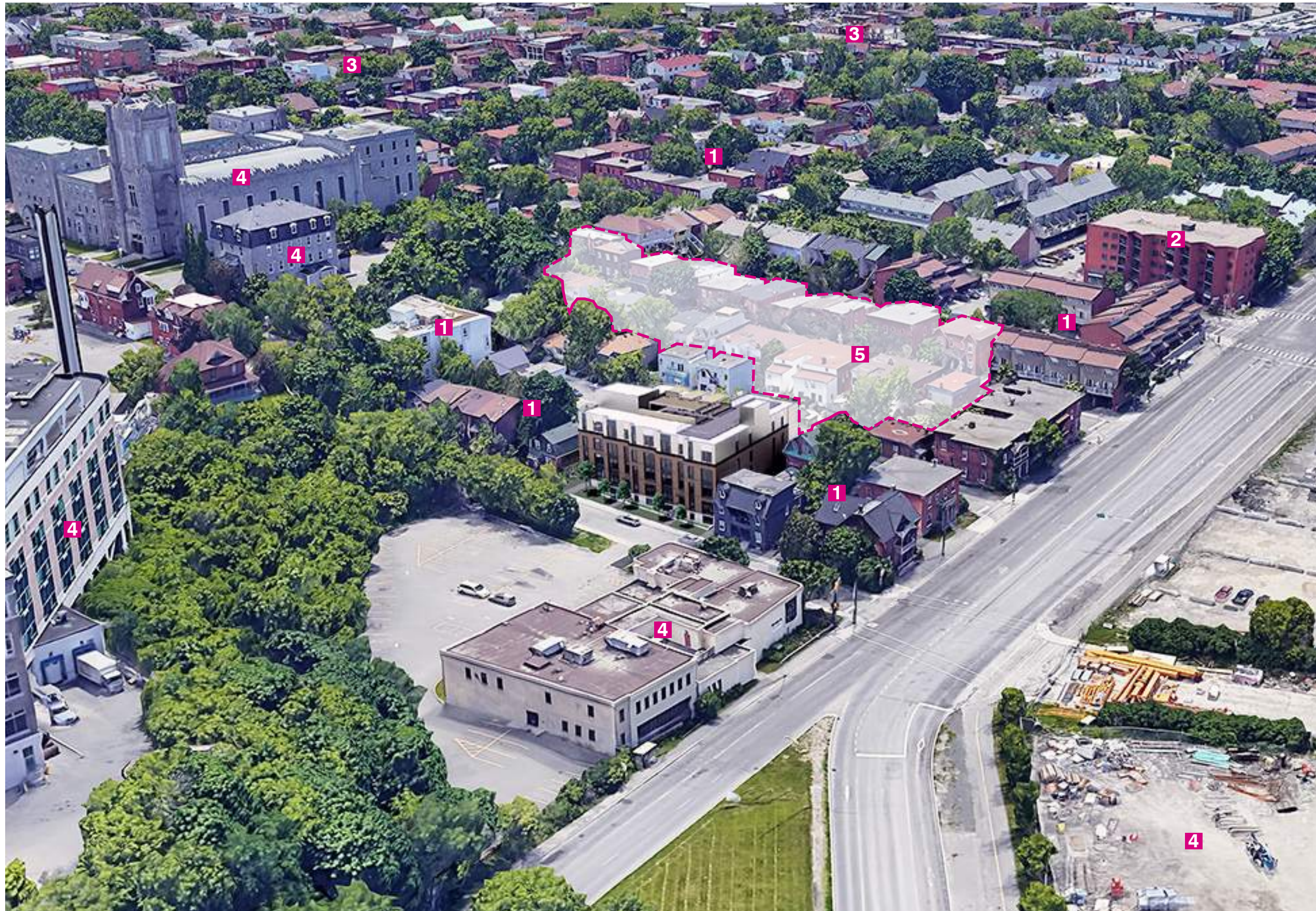
View Looking South
