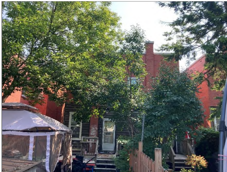
Photo 4 – Site Building B (west elevation).
