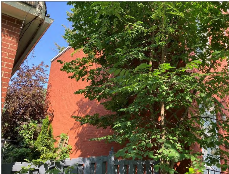
Photo 2 – Site Building B (south elevation).
