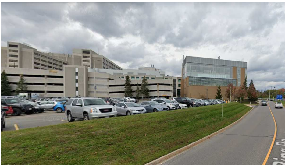
2. View of Ottawa Hospital from Ring Road (SE site boundary)
