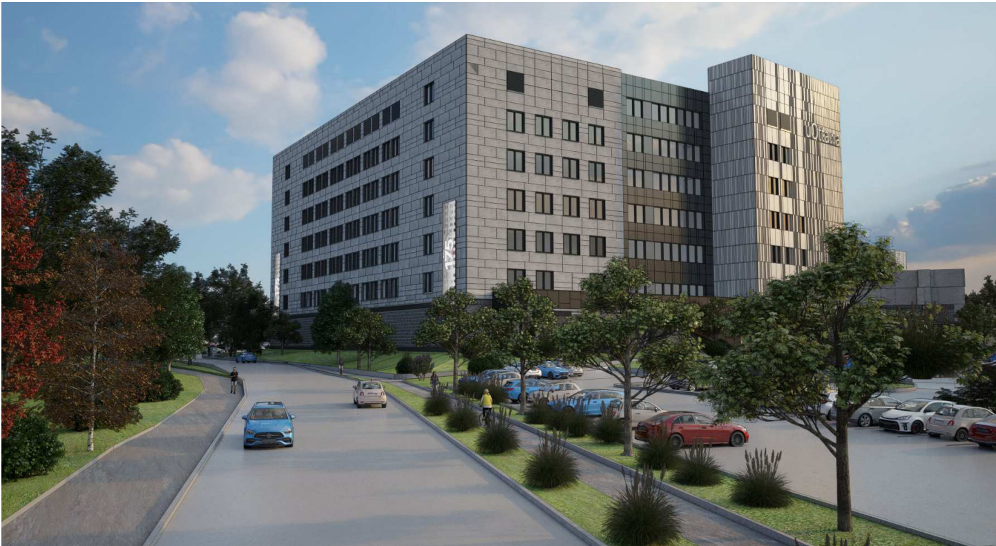
View of NW corner from Ring Road
