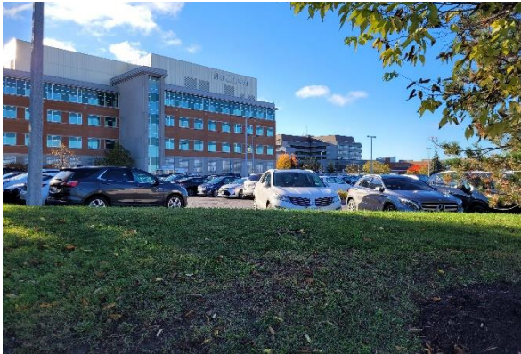
Figure 2-4: Site looking southwest towards Roger Guindon Hall
