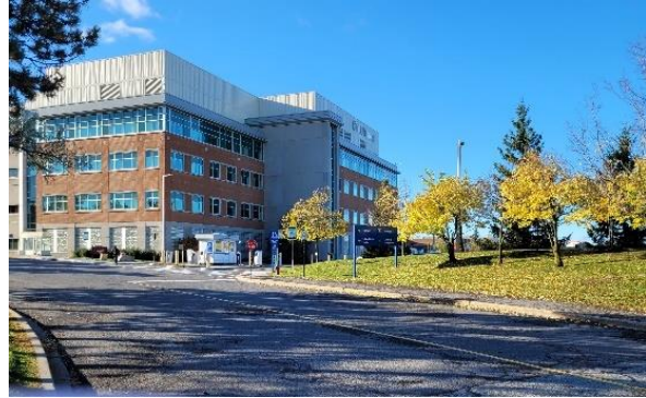
Figure 2-11: Site looking south towards Roger Guindon Hall
