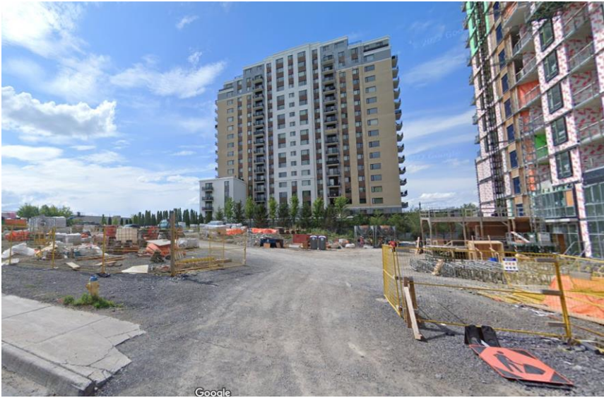
Existing site from Southeast corner.
