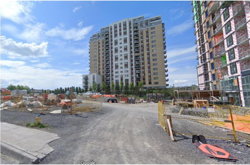
Existing site from Southeast corner.
