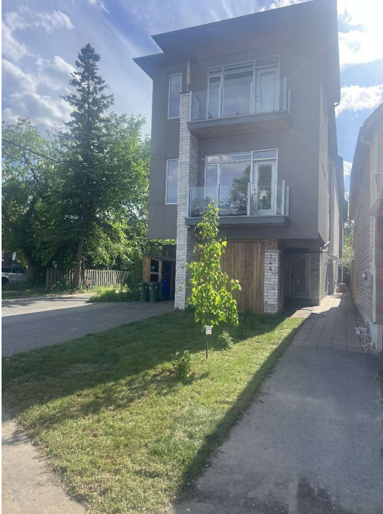
Existing front view
