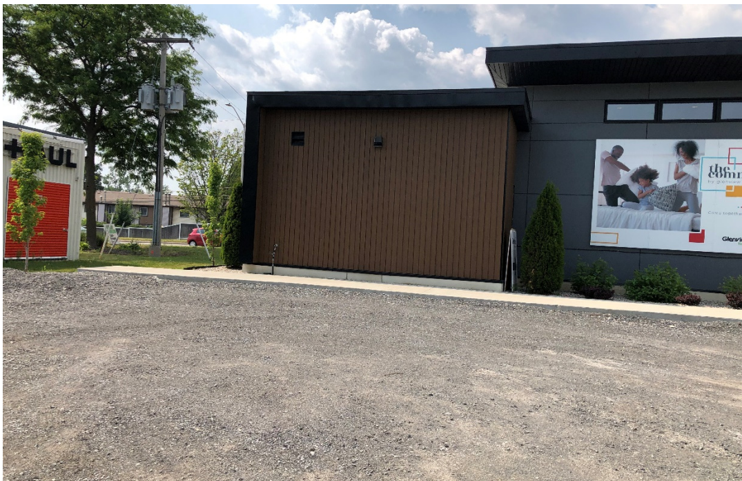
Photograph 2: View of south side of the building exterior.
