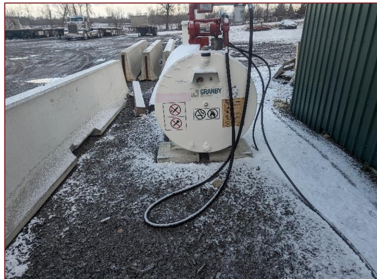
Photograph L18 – Looking north at one of the ASTs along the west building line of Structure 3 (Material Storage). The ASTs were in good working condition and there were no signs of spills, staining or odors were noted at this location.
