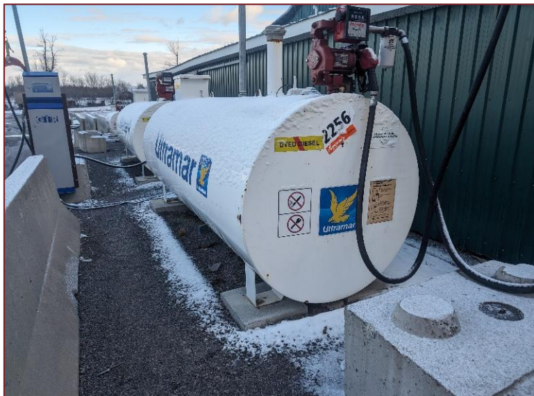
Photograph L17 – Looking north at the ASTs along the west building line of Structure 3 (Material Storage). The ASTs were in good working condition and there were no signs of spills, staining or odors were noted at this location.
