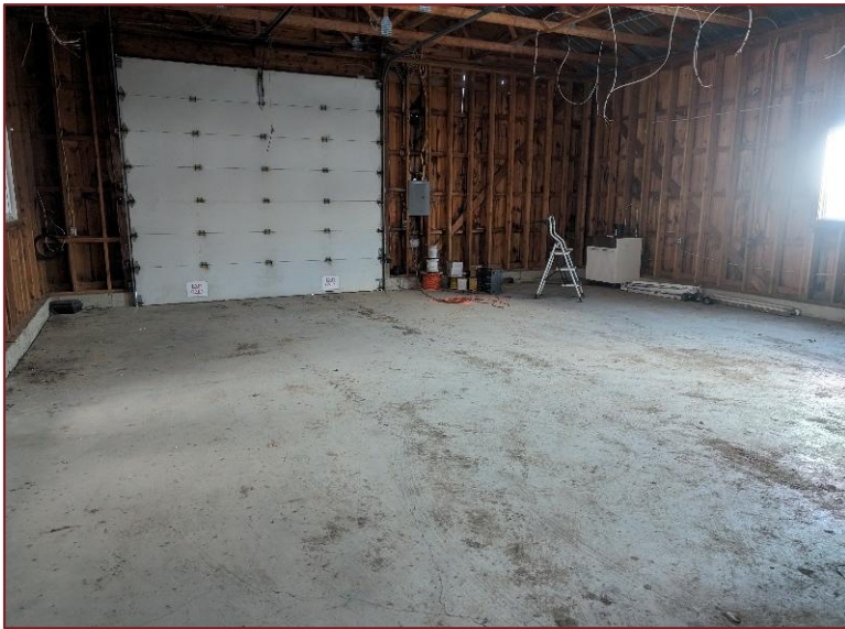
Photograph L21 – Looking north inside Structure 6 (Sales Shop). Concrete flooring was in a good shape with minimal cracking.
