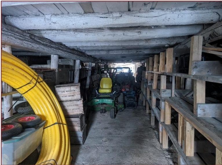
Photograph L15 – Looking north inside the Structure 3 (Material Storage). Concrete flooring was in a good shape with minimal cracking. No signs of spills, staining or odors were noted at this location.
