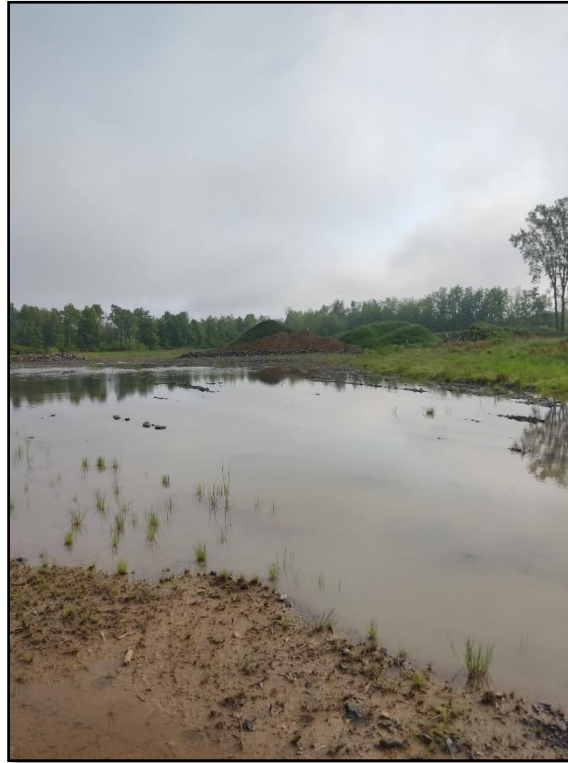
Figure 5: Area stripped of topsoil and now permanently wet with piles of topsoil in background (MH1284-D149).
