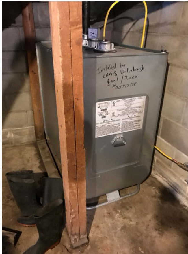
Photograph 28: Main house basement, heating oil tank
