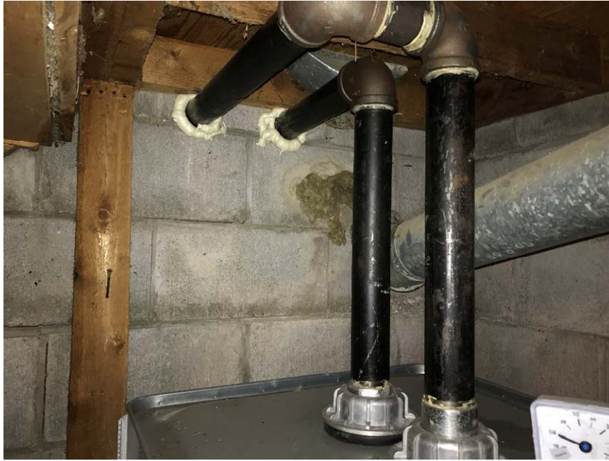
Photograph 29: Heating oil tank, fill and vent lines
