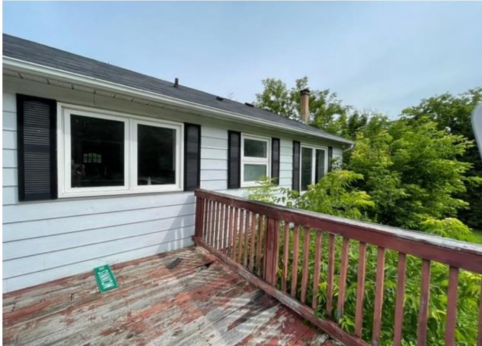
Photograph 6: View of the residential dwelling at 1458 Bankfield Road.
