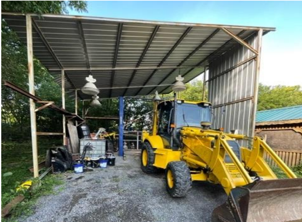
Photograph 13: View of the temporary/mobile service garage with above ground hoists at 1454 Bankfield Road.
