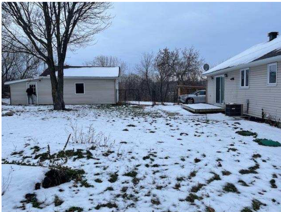
Photograph 18: View of the eastern side of 5485 Elijah Court, looking south.
