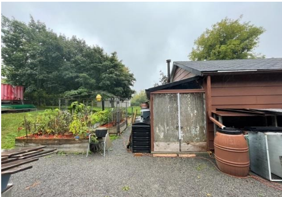
Photograph 16: View of the private garage/shed at 5479 Elijah Court.
