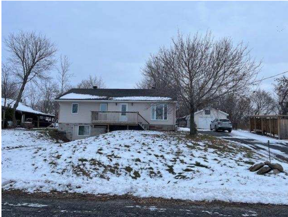
Photograph 17: View of the western side of 5485 Elijah Court, looking east.
