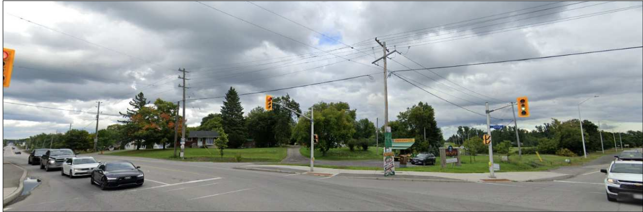
Figure 2: Subject Property from the intersection of Bankfield and Prince of Wales
