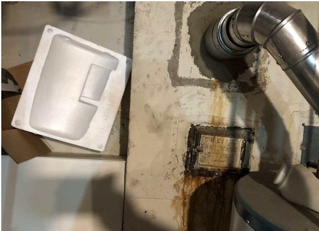
Photograph 2: Eastern portion of the basement, former chimney.
