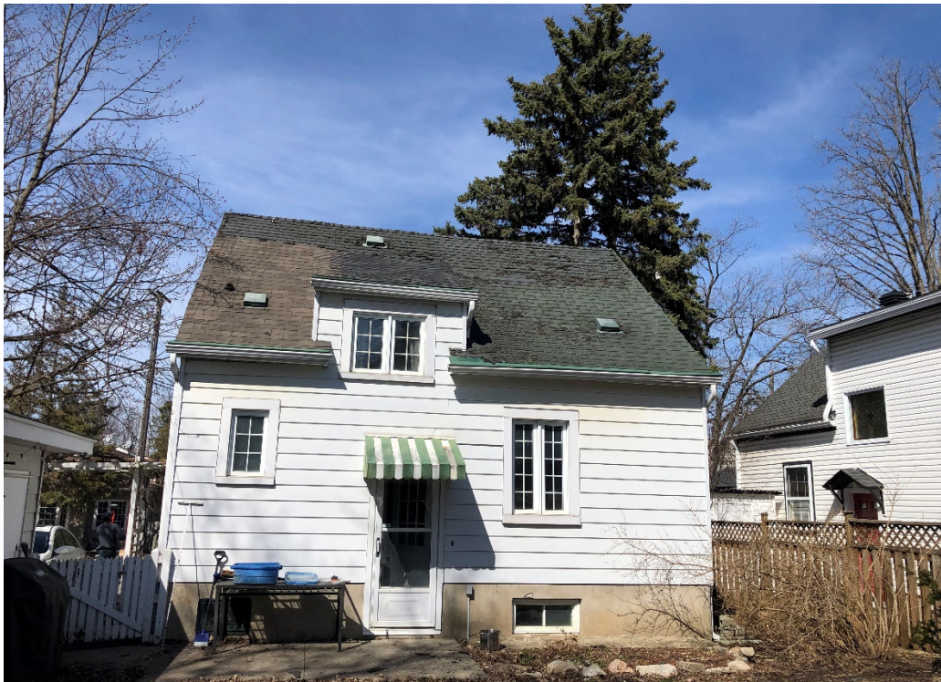
Photograph 4: View of the rear of the residential dwelling, looking north.
