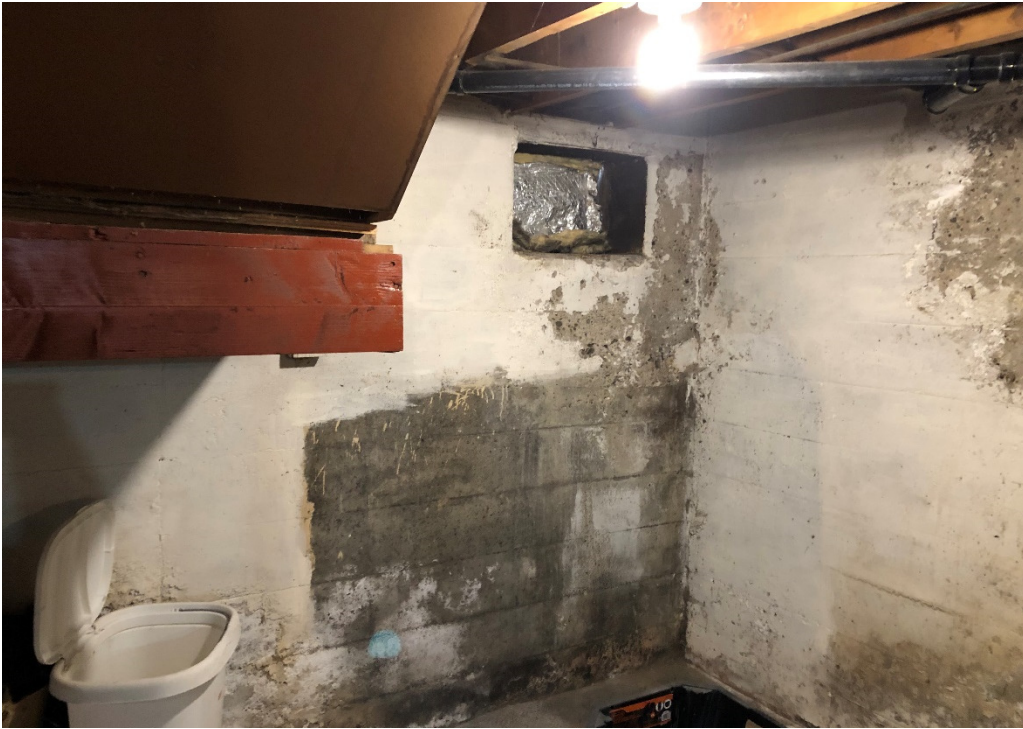
Photograph 1: Southwest corner of basement, former coal chute location.
