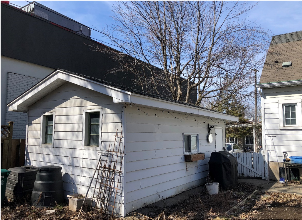
Photograph 5: View of the detached one-car garage, looking northwest.
