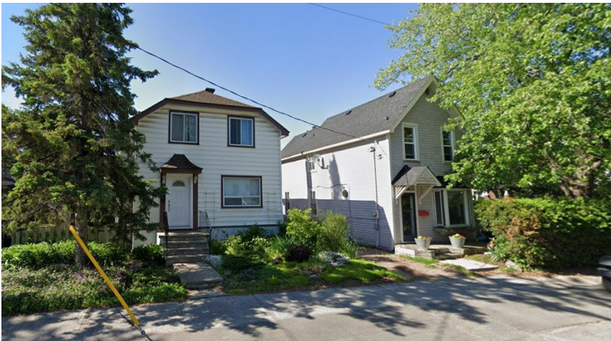
Figure 7 – Single Detached Dwellings to North of Subject Property
