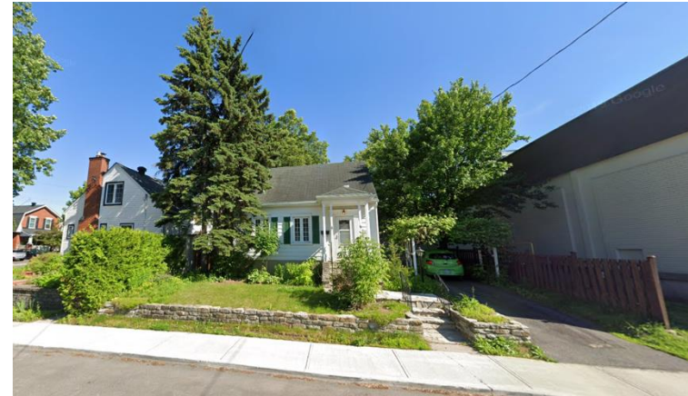
Figure 2 – Existing Street View of Subject Property
