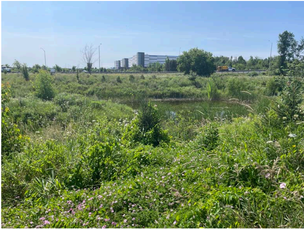
View of storm pond facing south
