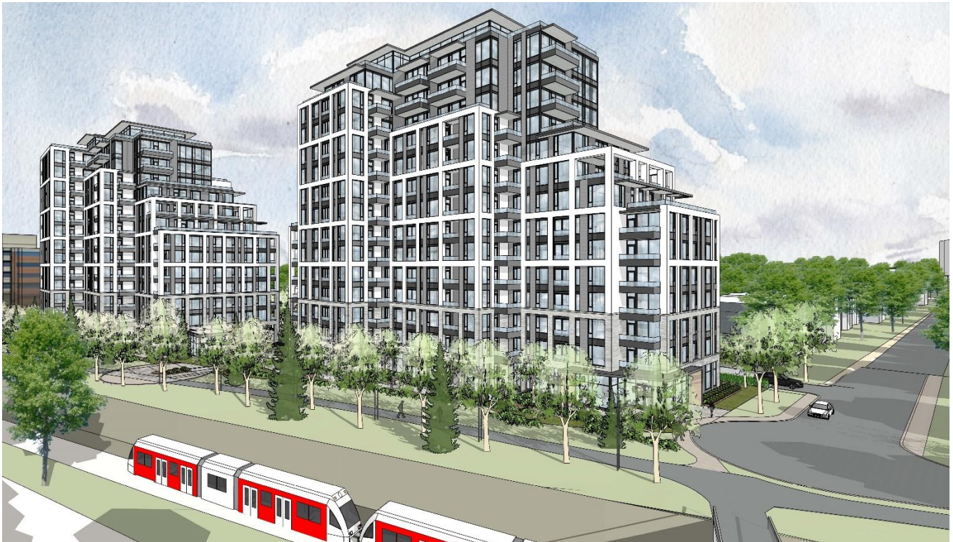
Figure 12: View from Workman Avenue. (Source: Hobin Architecture)
