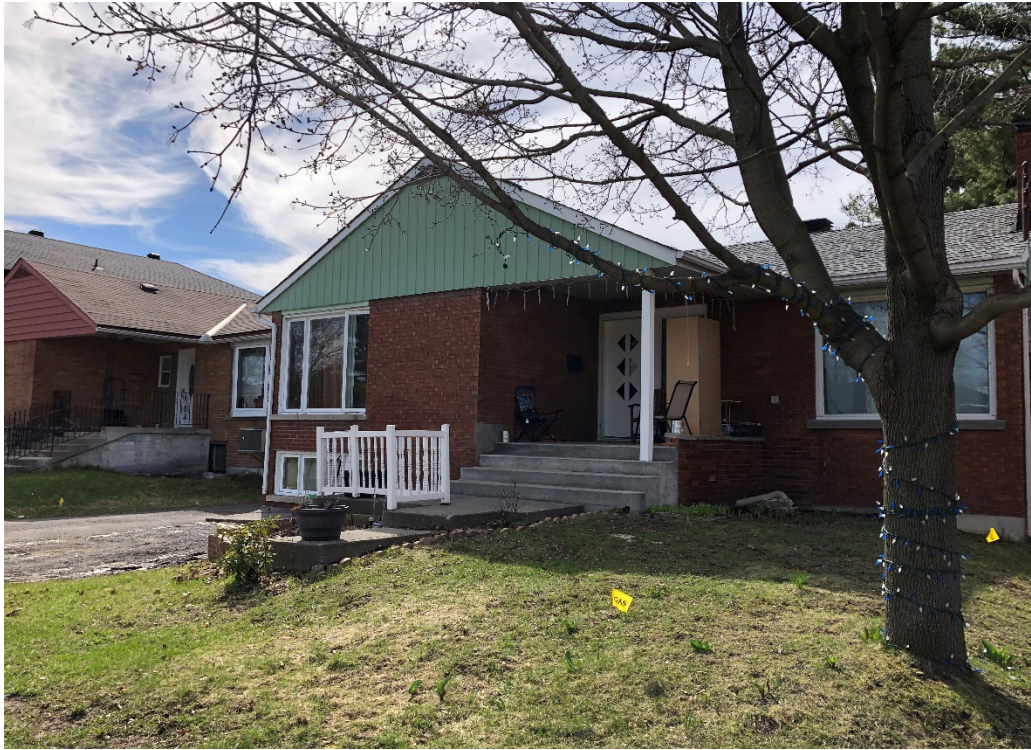
Photograph 5: View looking south from Donald Street, towards 308 Donald Street.
