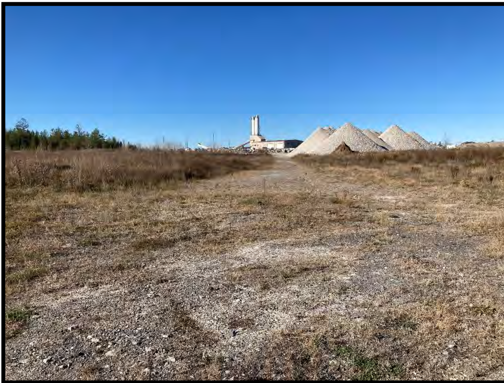
Figure 14: Portion of gravel roadway, stone piles, buildings of active quarry. (MH1141-D034)
