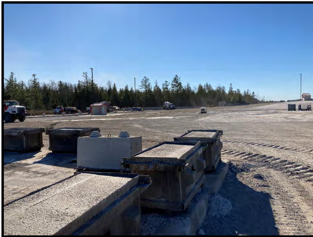
Figure 54: Active quarry, just north of the wooded marshland area. (MH1141-D130)
