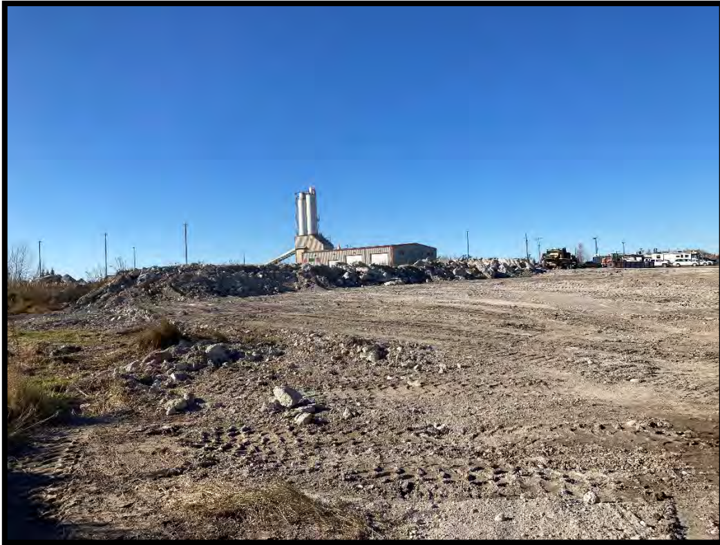
Figure 51: Work lot of active quarry in the northwest. (MH1141-D126)
