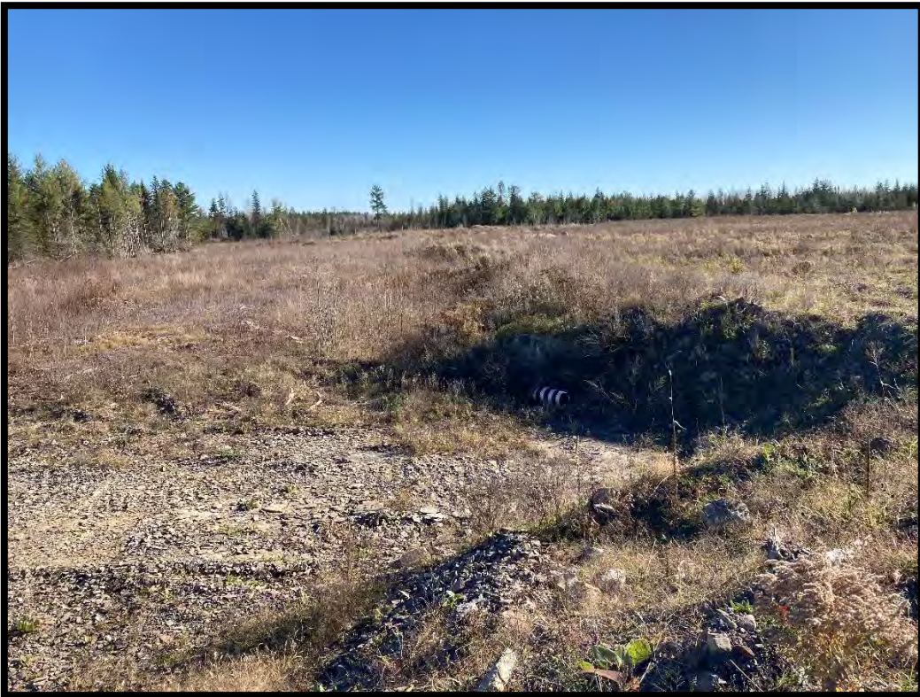
Figure 26: Edge of fill over bedrock and partially wet conditions in the south-eastern portion. (MH1141-D063)
