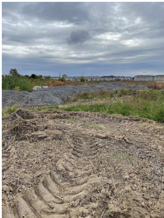
Photo 1: Aggregate piles south of parking area
