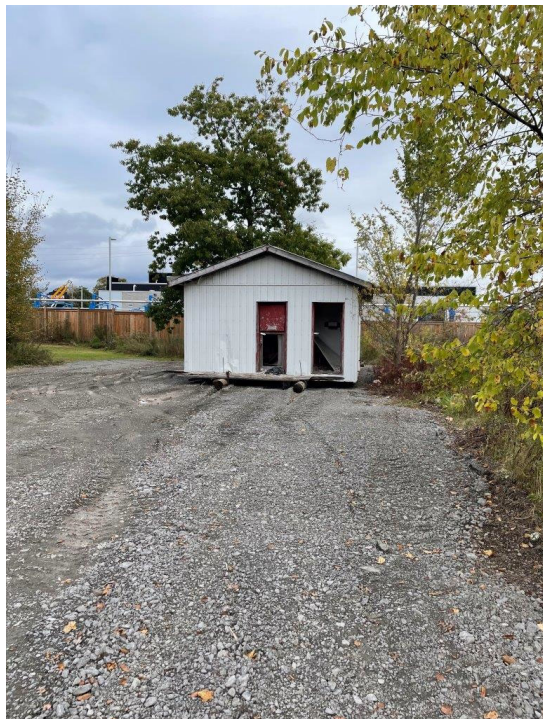
Photo 5: Mobile structure present in NE corner of parking area
