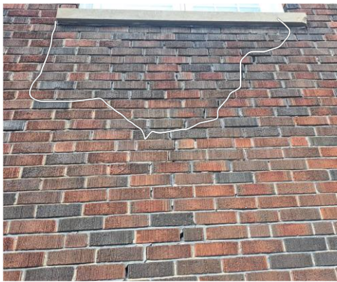
4. Staining of the brick under windows indicates long term water running down the face with cracking from the upper to the lower window.
