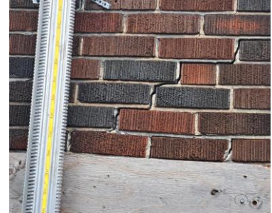
3. Stepped crack south end of east façade with vertical support lag bolted thro the wall.
