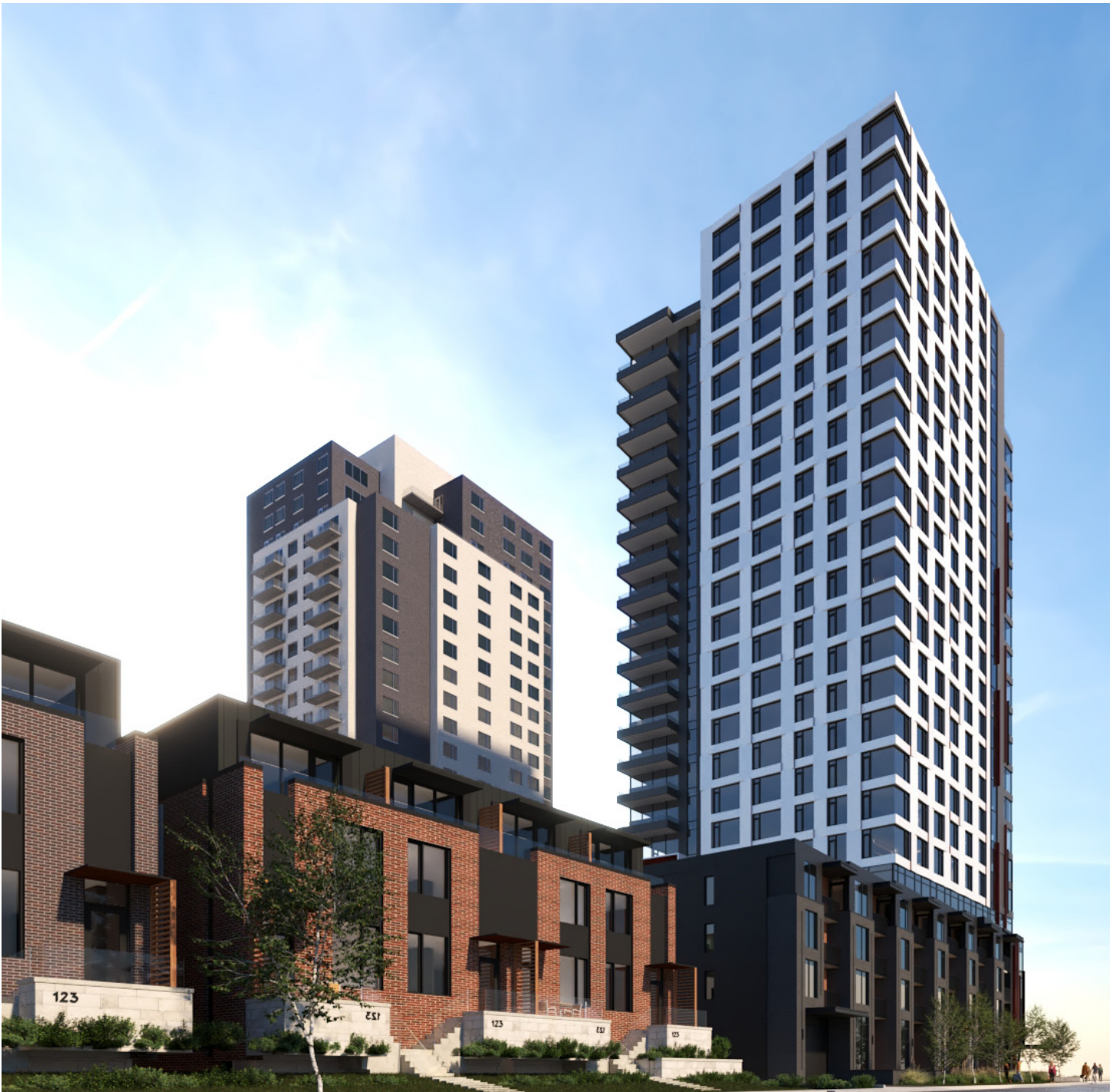
Figure 16.0 - View looking North along Clifton Road.
