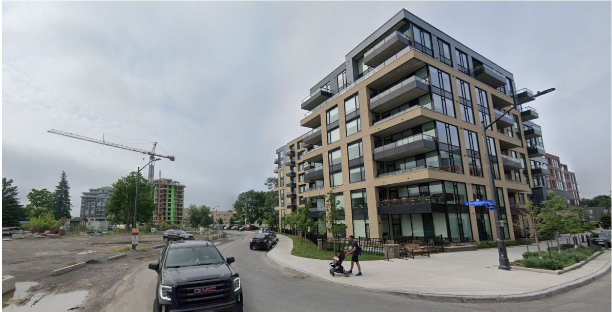
Image 5: Mid-rise development at Des Oblats Avenue and Deschâtelets Avenue intersection (looking south)
