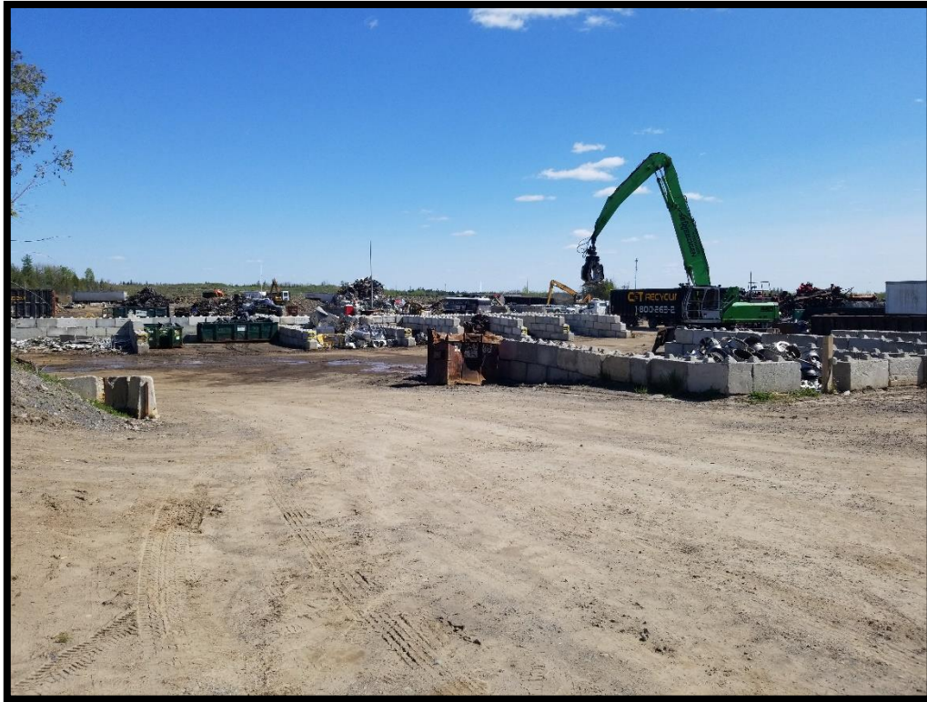
Figure 7: General conditions of northern recycling yard (MH1180-D069).
