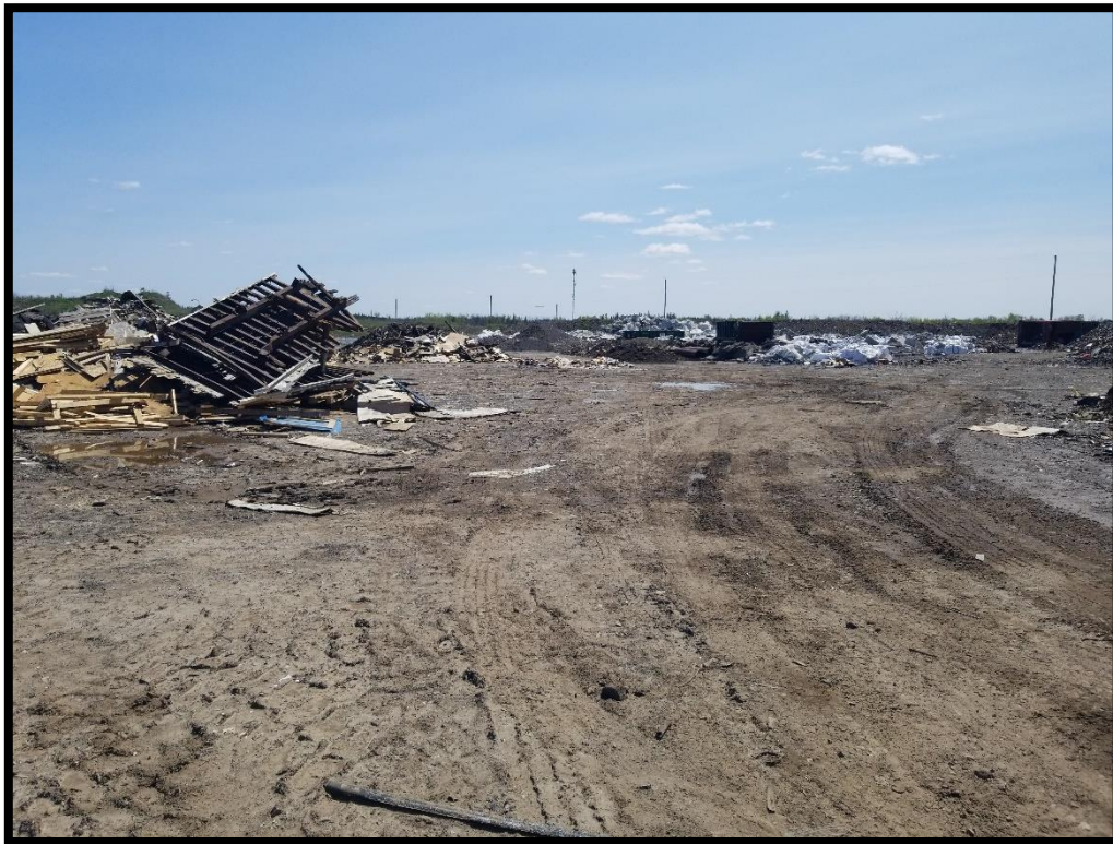
Figure 6: General conditions of southern recycling yard (MH1180-D020).
