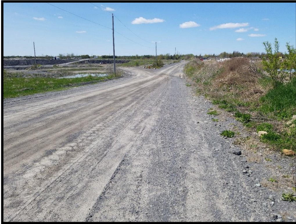
Figure 9: Gravel road running along western border (MH1180-D030).
