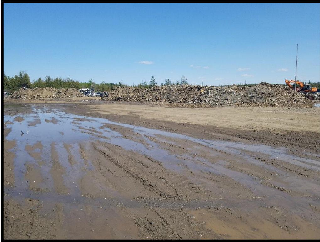
Figure 5: General conditions of northern recycling yard (MH1180-D018).
