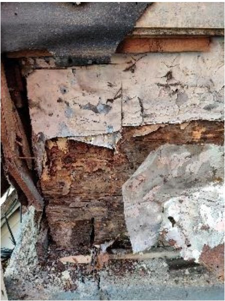
Figures 39 and 40 : The two views illustrate the multiple layers of finishes covering the squared timber, (tin panels insul-brick, ridged insulation, and vinyl siding.) Source David Yoo 2022.
