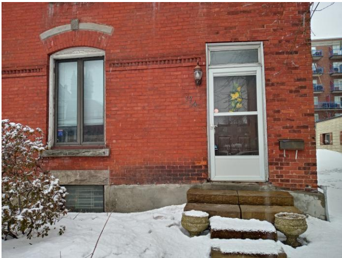
Figure 15 and 16: This collage of pictures documents the extensive alterations. Two views 1992 and 2022. 174 Murray (left) before the vinyl siding being removed and rehabilitated front. Note the different brick at the corner (both size and colour consistency) and the lack of corbelled banding and the transom treatment.
