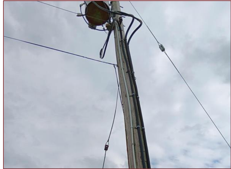
Photograph L14 – Looking north, up the pole. An electrical transformer on the pole with no staining seen on the wood below it..
