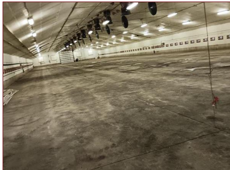
Photograph L6– Looking west inside the barn. Slab floor on grade. Venting overhead and vent windows along wall. Some staining from agricultural practices.
