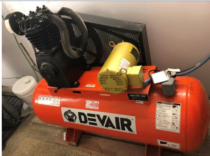
Picture 5 – Air Compressor Within 2 nd Floor Mechanical Room of Office Building
