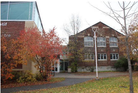
Photo 13 Plant Recreation Centre south entrance, looking northwest
