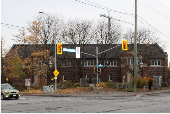
Photo 9 Plant Bath looking southwest
