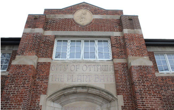
Photo 11 Plant Bath northeast former entrance
