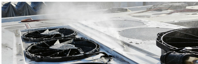
figure 5-38 Schematic Diagram of Maintenance Process with High-pressure Water Gun
