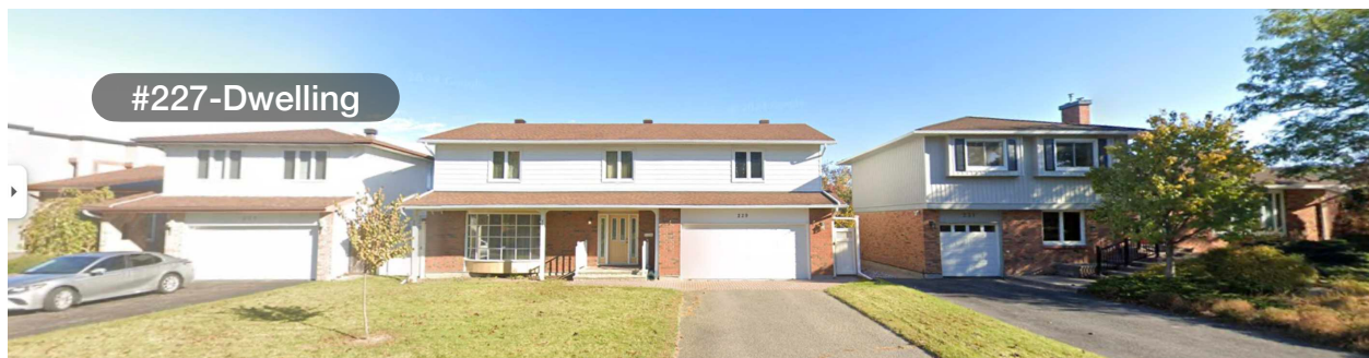
Figure 3: Existing dwelling at 227 McClellan Road to be severed
