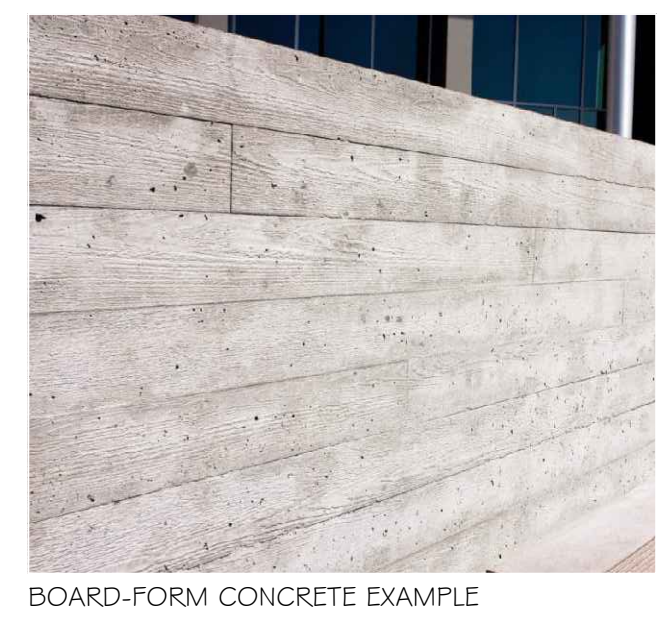
BOARD-FORM CONCRETE EXAMPLE
