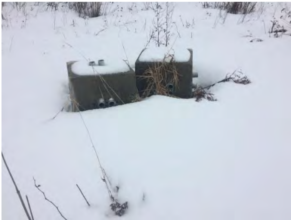
Photo 12: Concrete blocks located on the eastern portion of the Site just south of the dirt and gravel road.
