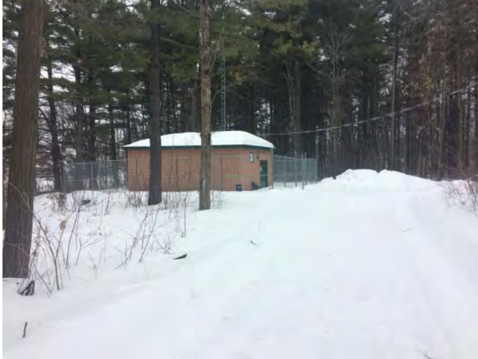
Photo 19: Photo of the pump house located within a treed area immediately west of the Site.
