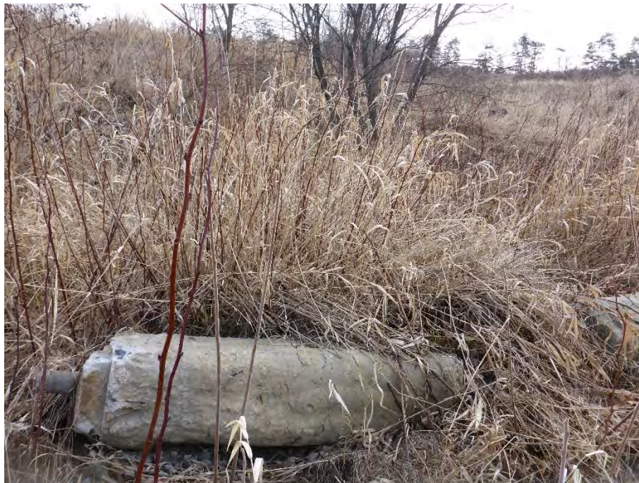
Image 4: Cement block with metal bar located north of the gravel path, view northeast.
