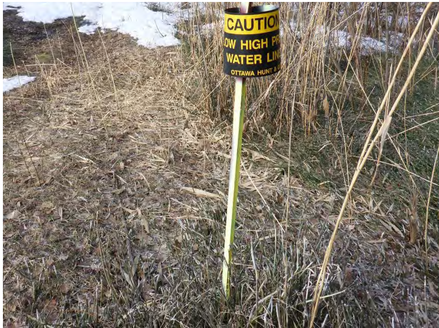
Image 5: Sign showing the location of a high pressure water line in the northern portion of the study area, view southwest. The signs indicated lines were running southwest to northeast along the western border of the study area and east to west along the northern border.
