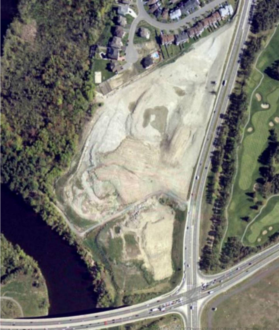
Figure 15: Aerial view, 2002, of the development site. (Source: EMaps, City of Ottawa, online at http://maps.ottawa.ca/geoOttawa/ . Annotated by Contentworks.)
