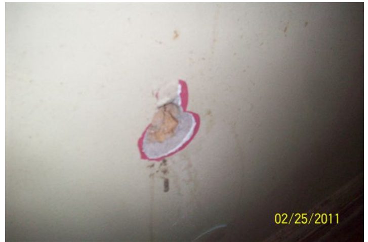
Photo No. 2 – Wall Plaster, Sample Group 72-AS-022511-02
