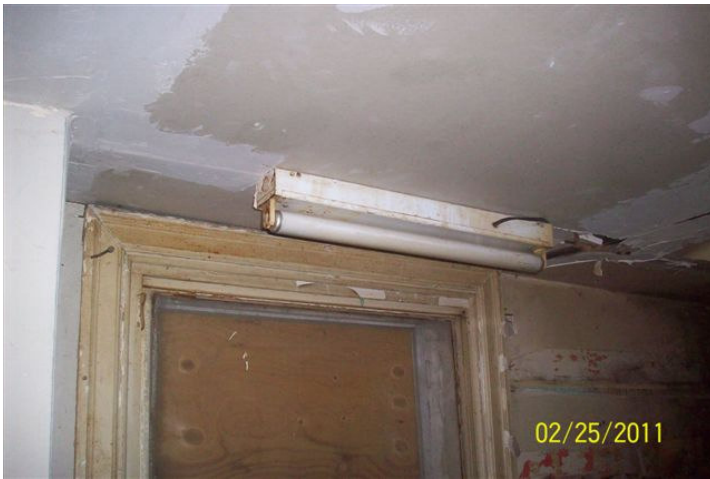
Photo No. 7 – Potential PCB containing ballast and mercury vapour containing fluorescent tube.
