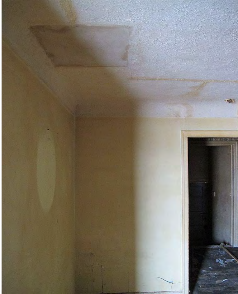
21 living room ceiling
