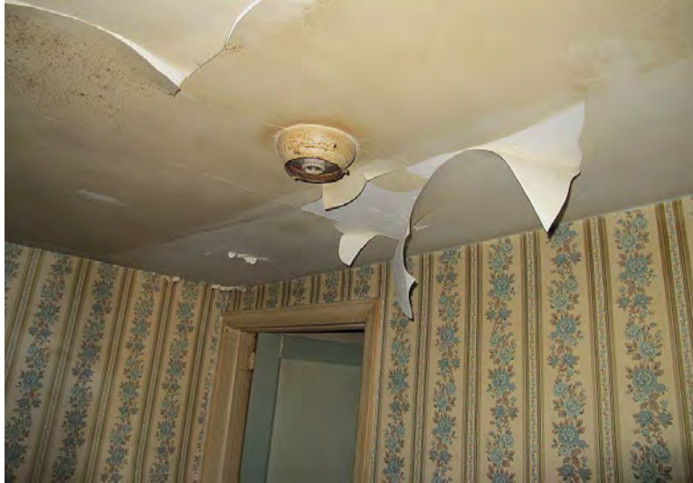
dining room ceiling
