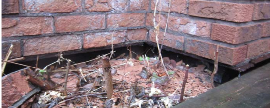
Photo 2 – Base of Brick Wall & Support Angle
