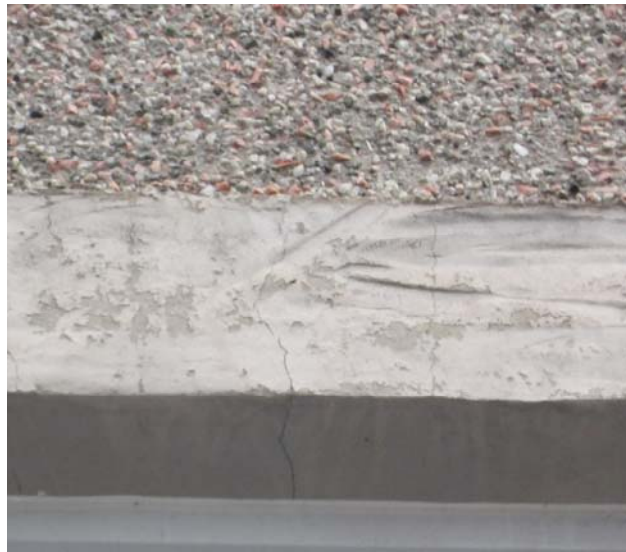
Photo 3 - Cracked Lintels
