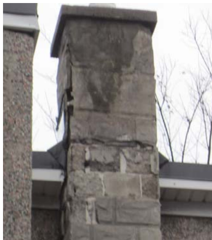
Photo 1 - Damaged Chimney
