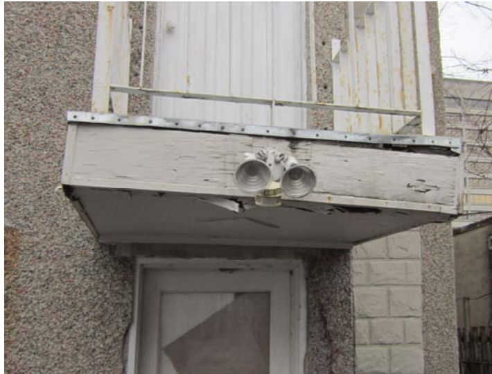
Photo 2 - Rear Door Awning/Balcony
