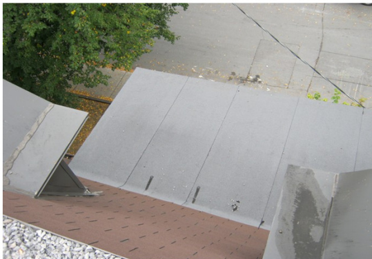
Photo: F01085_B3010 Roof Coverings - Mod Bit_1
