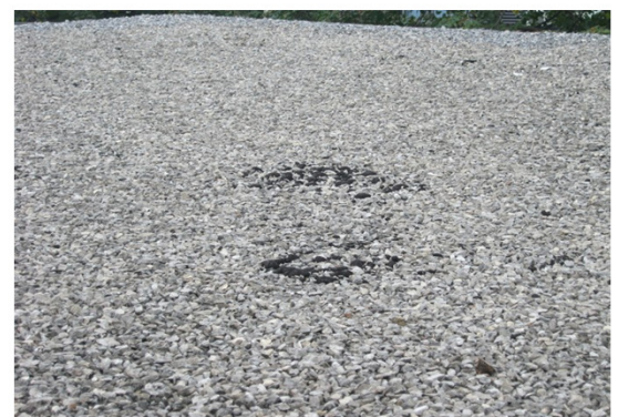
Photo: F01085_B3010 Roof Coverings - BUR_2
