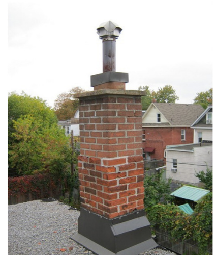
Photo: F01085_B201001 Exterior Closure - Brick - Chimney Sept 2011_2
