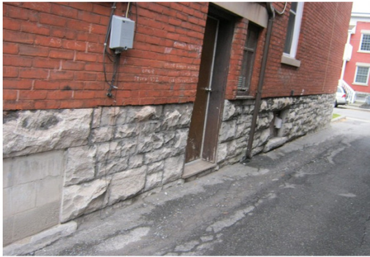
Photo: F01085_A10 Foundations_Sept 2011_1
