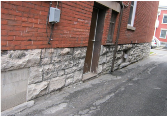
Photo: F01085_GA10 Foundations_Sept 2011_1
