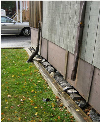
Photo: F01085_B3010 Roof Coverings - Roof Drains - Downpouts BUR_1
