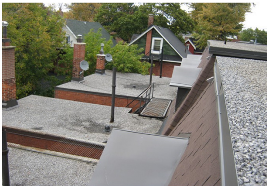
Photo: F01085_B3010 Roof Coverings - BUR_1
