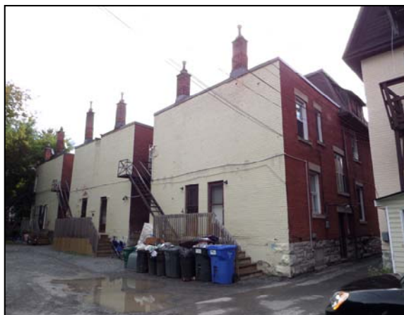
Photograph 1 – 143-153 Arlington Ave., Ottawa, ON, showing the Northern (rear) additions.
