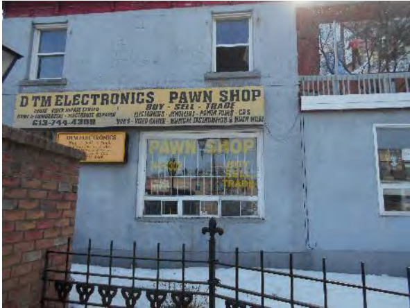
Partial view of the north elevation of the Site Building.
