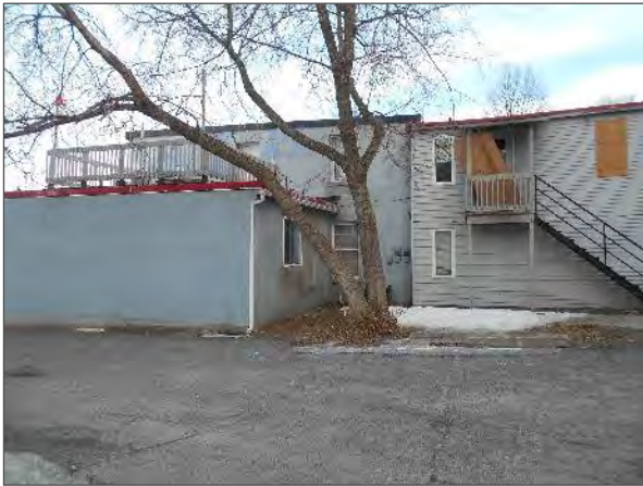
View of the west elevation of the Site Building.
