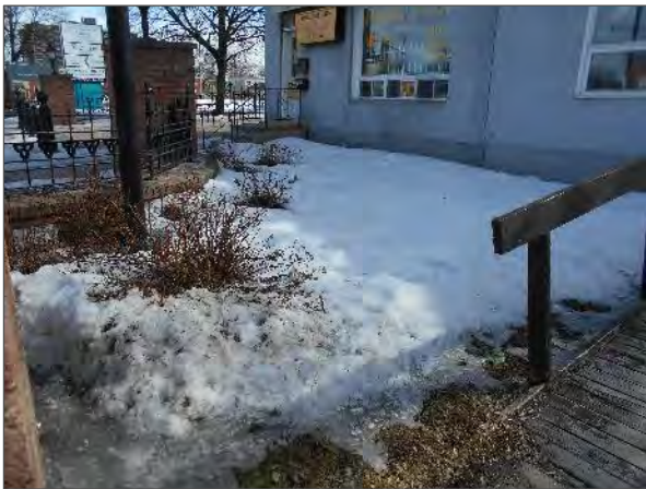
General view of the Site features on the north portion of the Site.
