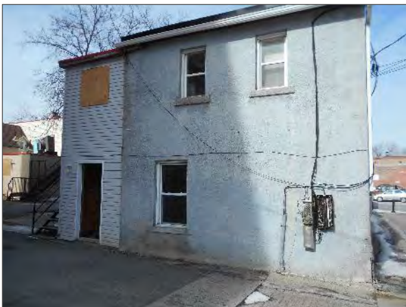
View of the south elevation of the Site Building.
