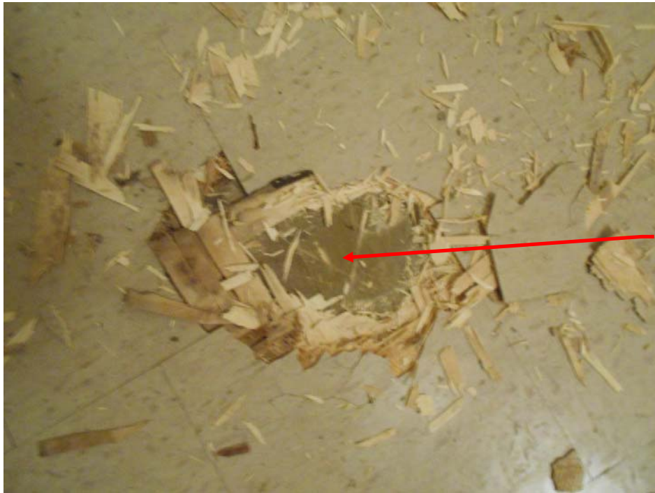
Photo 13 – South (Gladstone) Building | VFT – olive grey tiles under laminate floor
