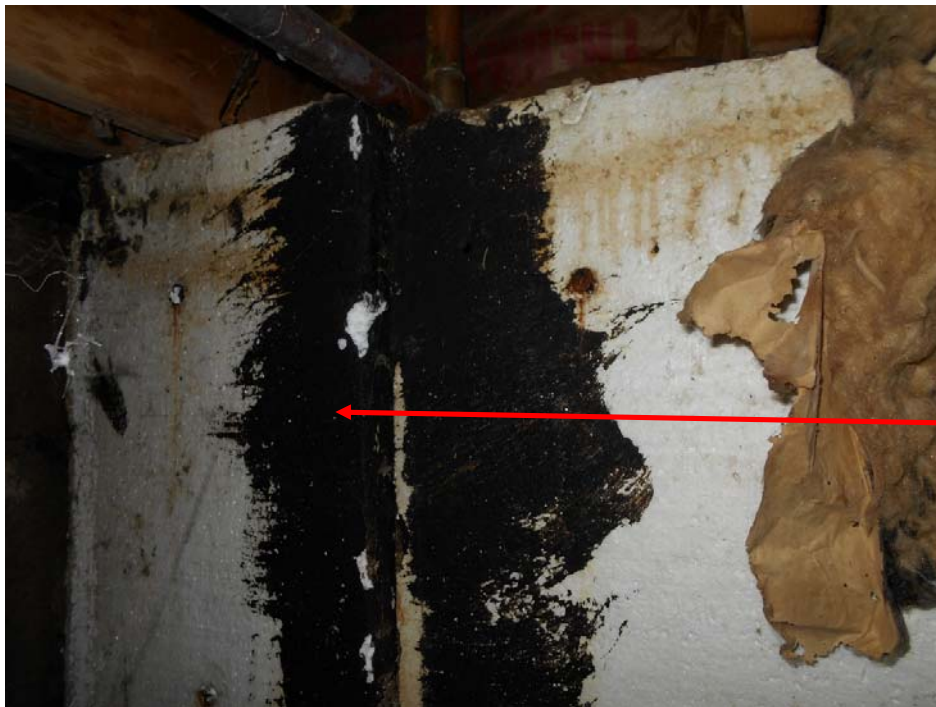
Photo 8 – West (Rochester) Building | black tar damp proofing holding Styrofoam to walls
