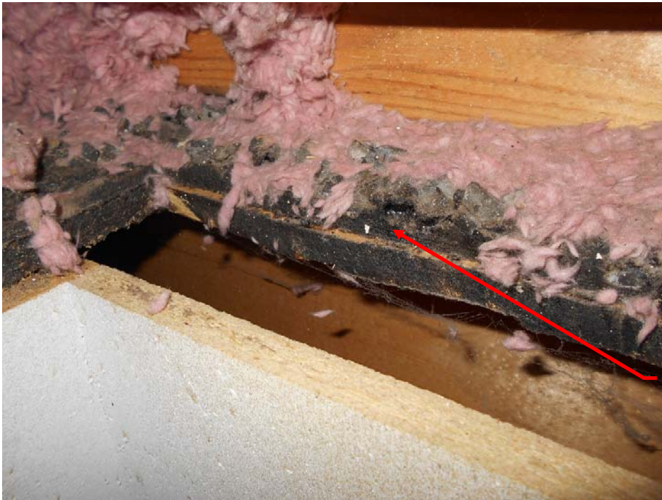
Photo 9 – South (Gladstone) Building | tar and gravel flat roof forming attic floor
