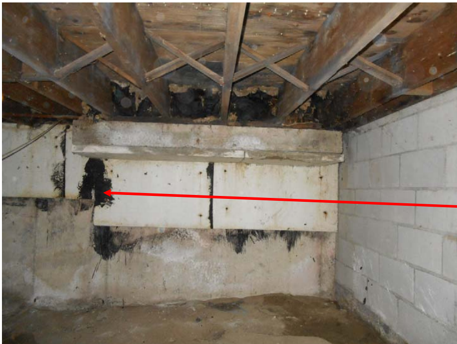
Photo 10 – South (Gladstone) Building | tar damp proofing used to attach Styrofoam panels to crawlspace walls
