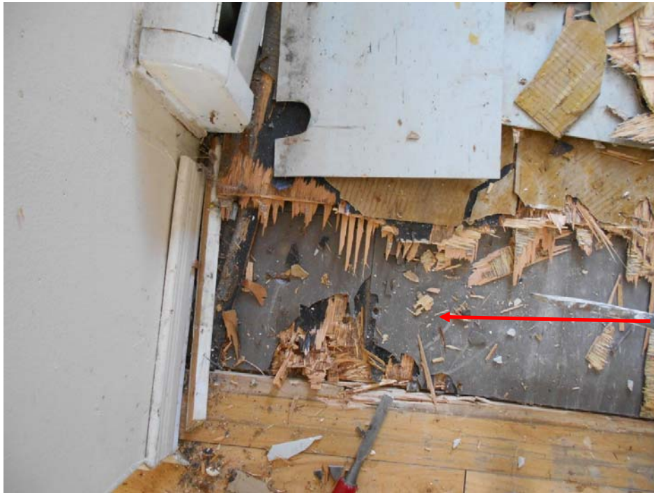
Photo 5 – North (Balsam) Building | VFT – 8"x8", brown with white streaks
