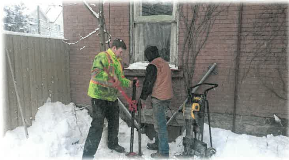
Photograph 4: Installation of MW1 by CM3 in December 2016.
