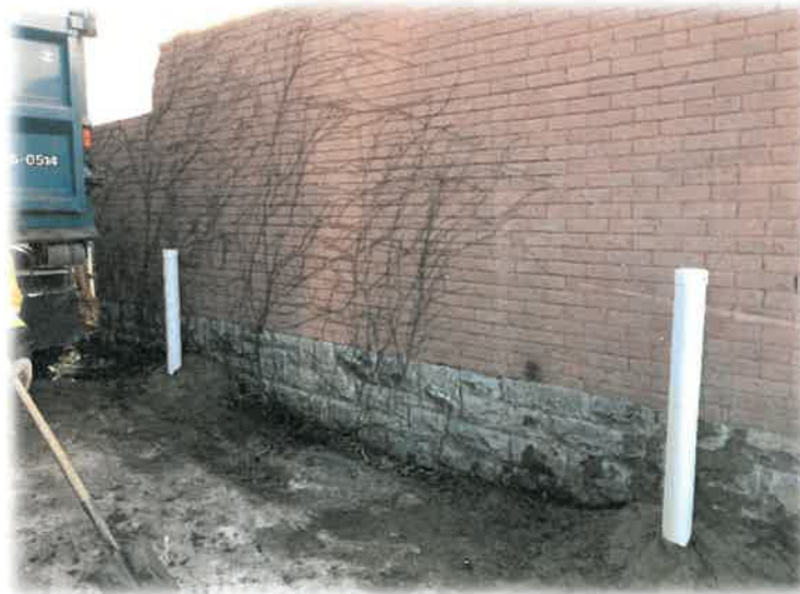
Photograph 8: View of east side of 22 Hawthorne at BH 14 and BH15.
