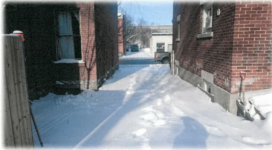
Photograph 3: View of shared laneway and east side 22 Hawthorne and west side of 24 Hawthorne.
