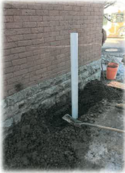
Photograph 7: East side of 22 Hawthorne and hydro-vacuumed hole for BH14.
