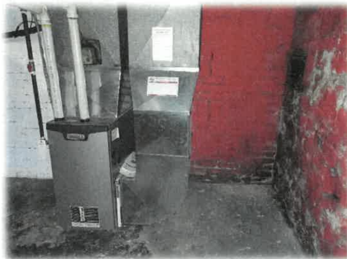
Photograph 10: View of interior of basement 20 Hawthorne.
