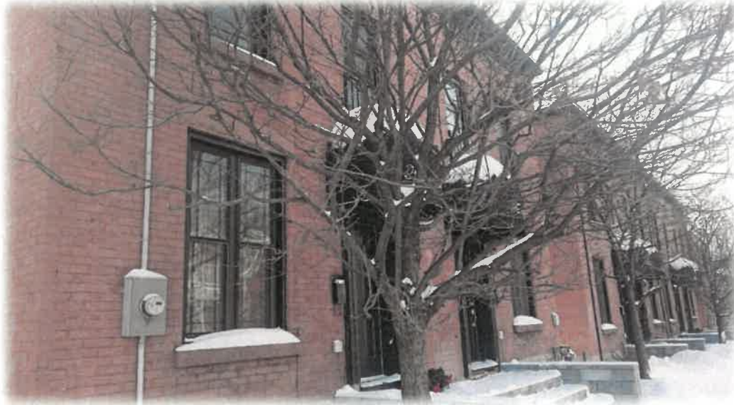
Photograph 1: View front of 20 and 22 Hawthorne on property looking south west.
