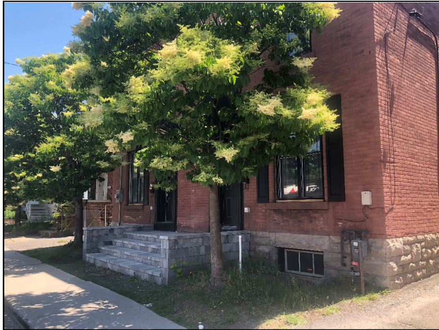
Photograph 1: 20-22 Hawthorne Avenue Main Entrances, Looking South-East
