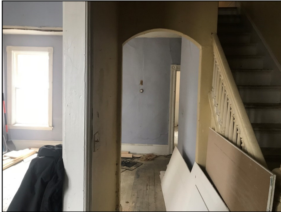
Photograph 9: Typical main interior finishes for 22 Hawthorne
