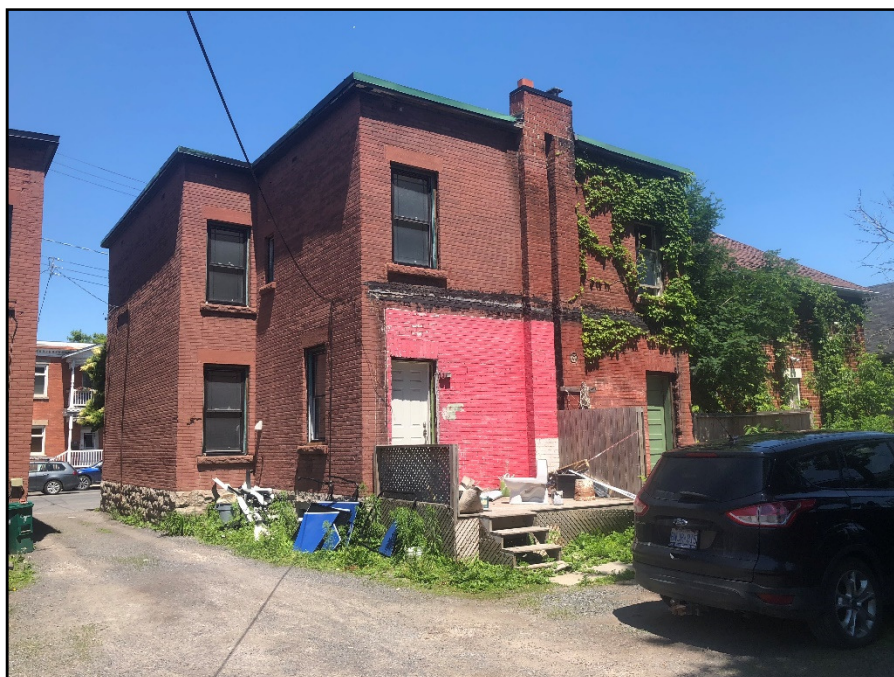
Photograph 4: East wall of 20 Hawthorne and south wall of 20-22 Hawthorne, looking north-east
