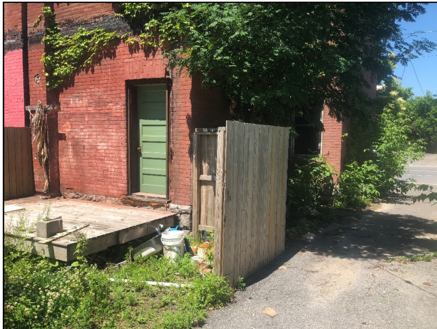
Photograph 7: View of south and east wall of 22 Hawthorne
