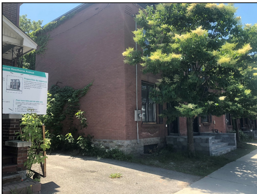
Photograph 6: Looking south-west at front wall and east wall of 22 Hawthorne
