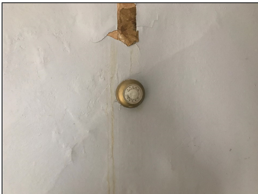
Photograph 12: Thermostat on main level in 22 Hawthorne
