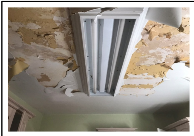
Photograph 3: Mercury containing fluorescent light tubes located throughout residence.
