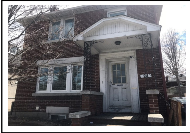
Photograph 1: 24 Hawthorne Avenue – Exterior
