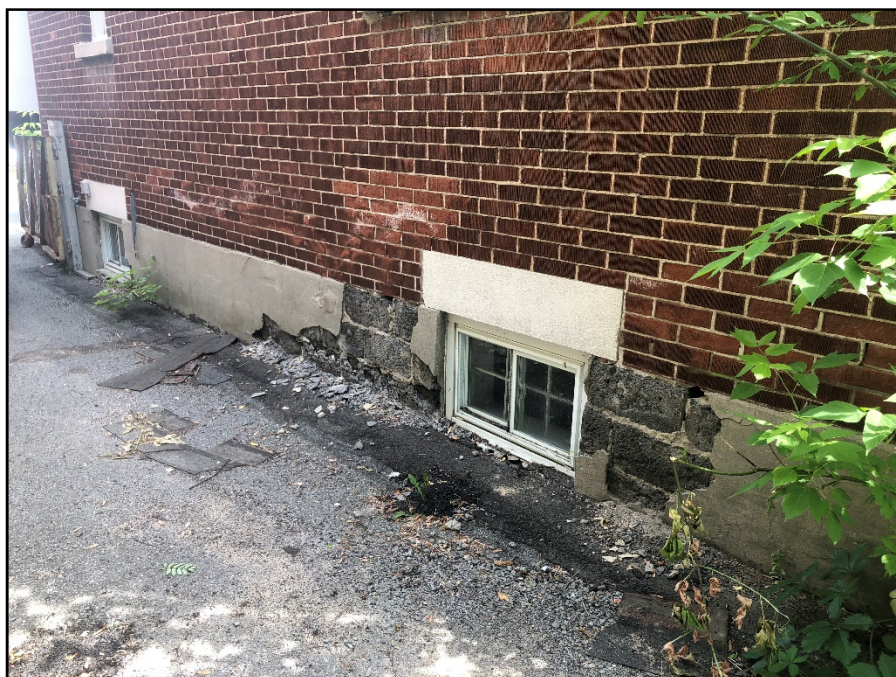
Photograph 4: West wall of 24 Hawthorne, looking North-East
