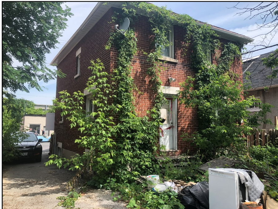
Photograph 5: Exterior view of south and east wall, looking north
