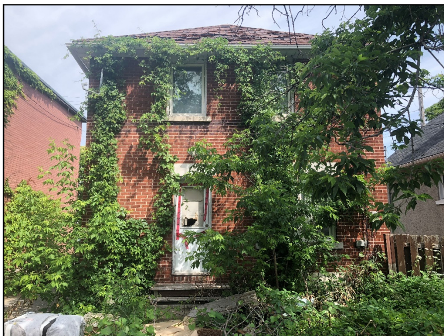
Photograph 6: Looking North at South wall and roof
