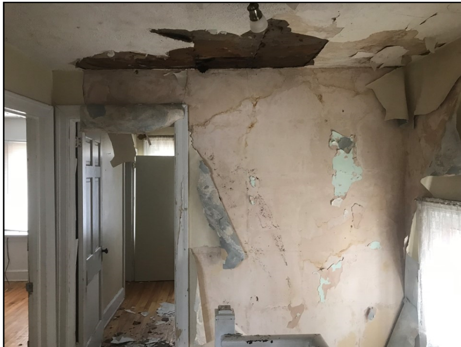
Photograph 9: Typical upper interior finishes
