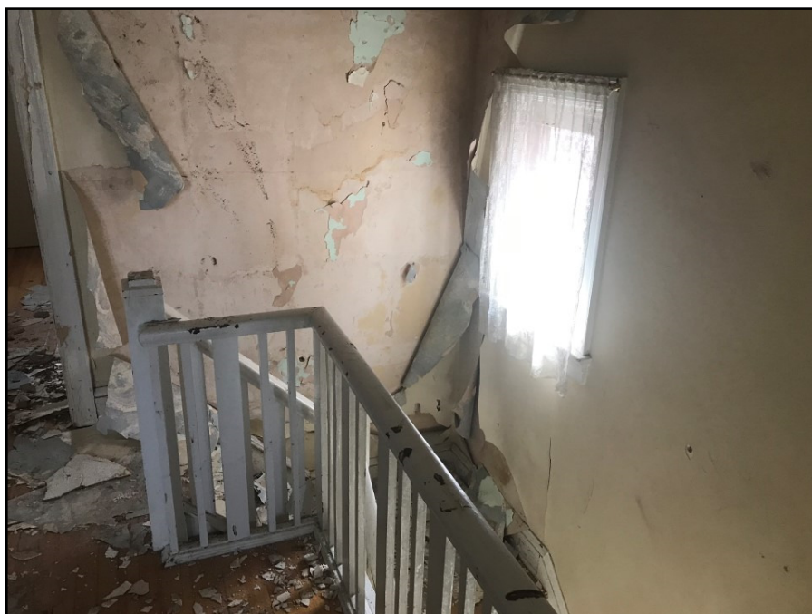
Photograph 10: Stairwell leading to ground level of home
