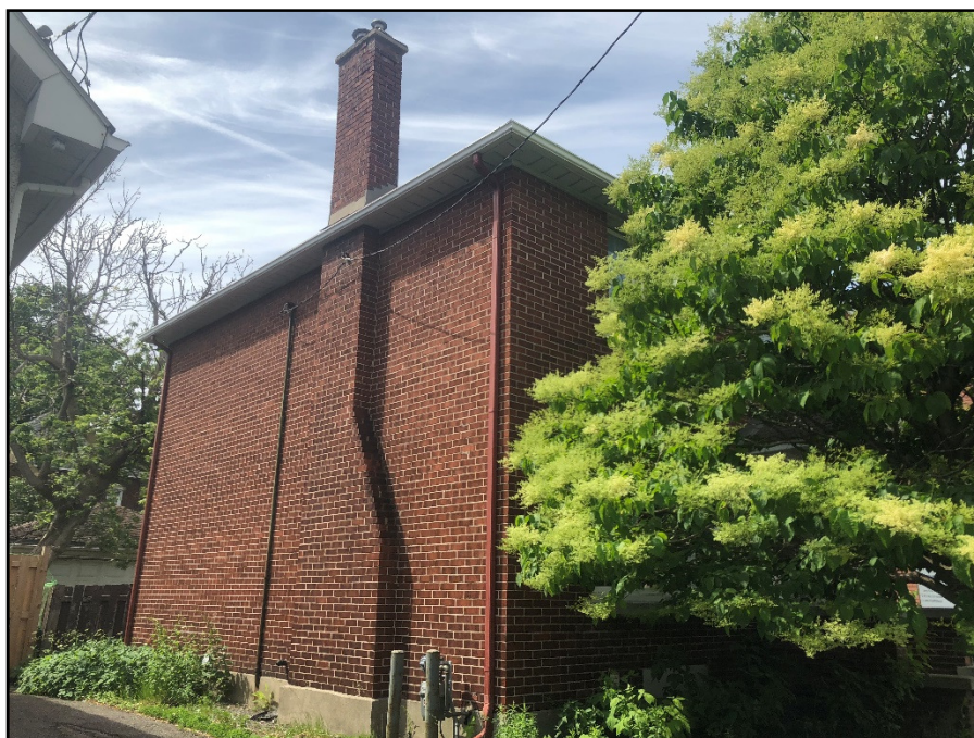
Photograph 2: East side of 24 Hawthorne, Looking South-West
