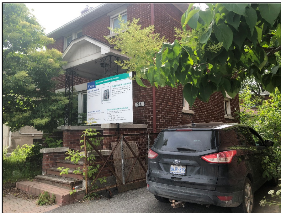
Photograph 1: 24 Hawthorne Avenue Main Entrance, Looking South-East
