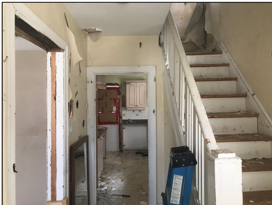
Photograph 12: Main level with view of kitchen
