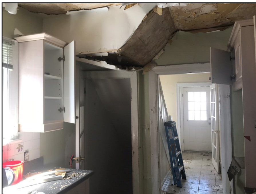
Photograph 14: View from kitchen of front door with stairwell on the right
